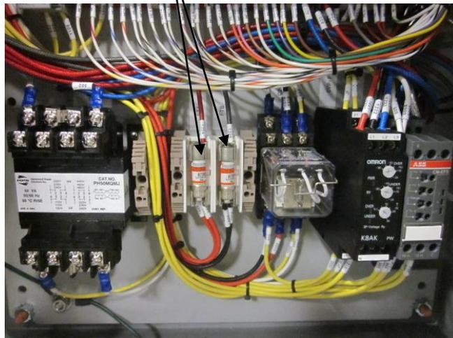
Figure 7a. Control Fuses (Operator Enclosure)
