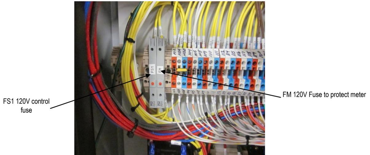
**Figure 7b. Control Fuses (Operator Enclosure)**
