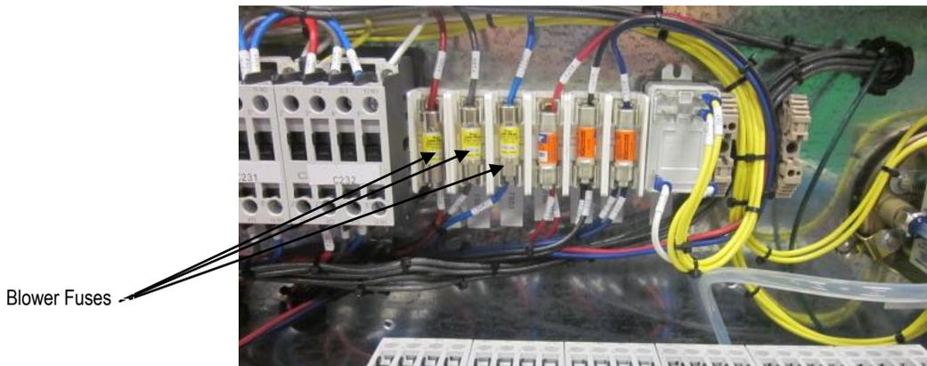
**Figure 5 Blower Fuses in the Main Panel**
